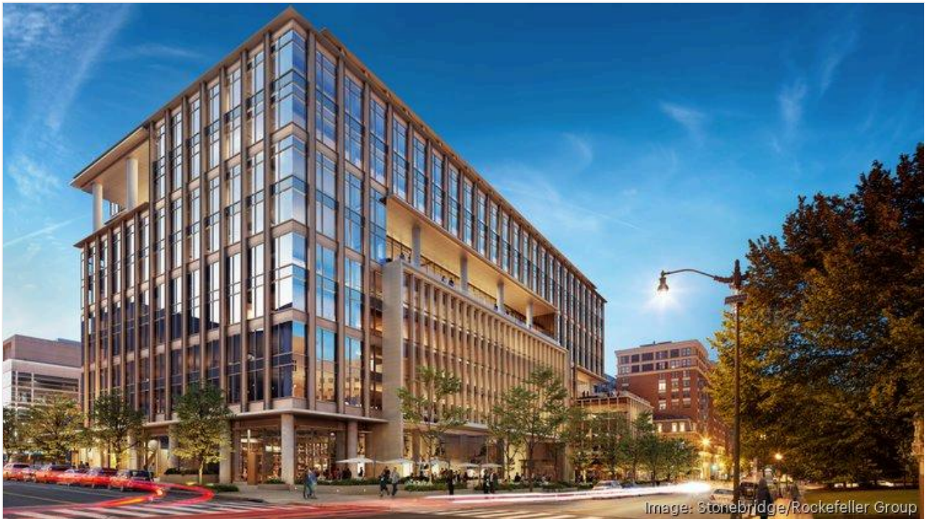
AFTER: 600 Fifth St. NW as it will look when the project is completed in 2026.
